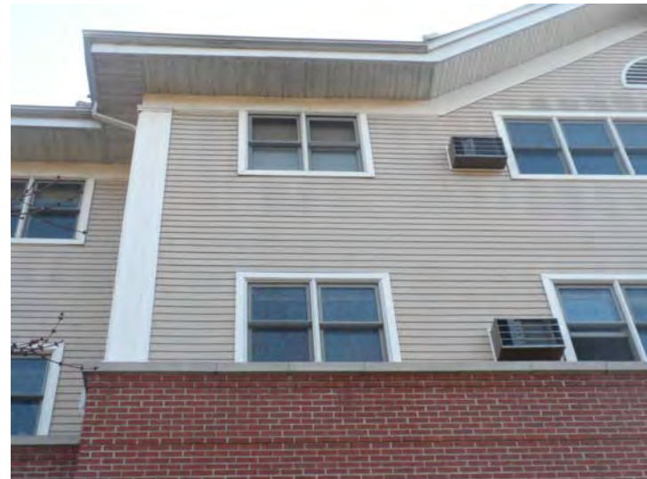
Typical siding and brick condition; good overall condition
