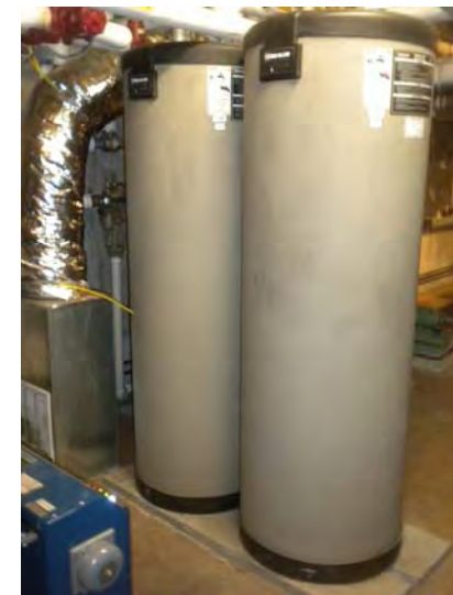
View of the two indirect domestic hot water storage tanks
