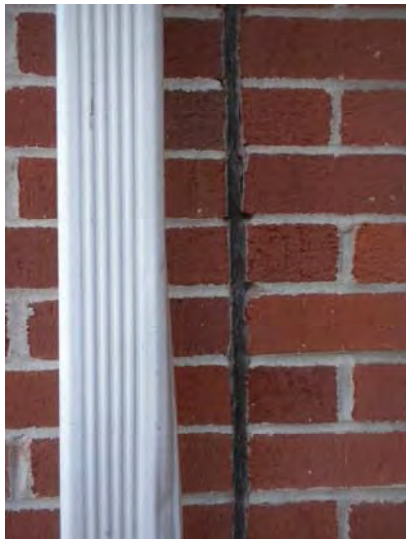
Cracking/hard expansion joint caulking
