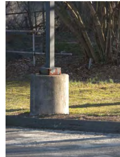
Example of rusted base to a pole mounted light fixture
