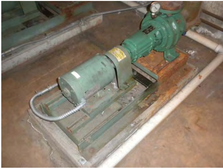
One of two heating water circulator pumps
