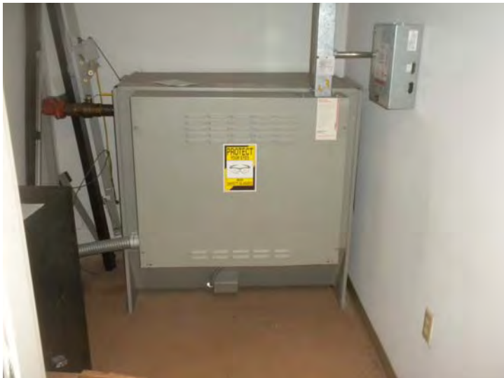
Hydraulic elevator package
