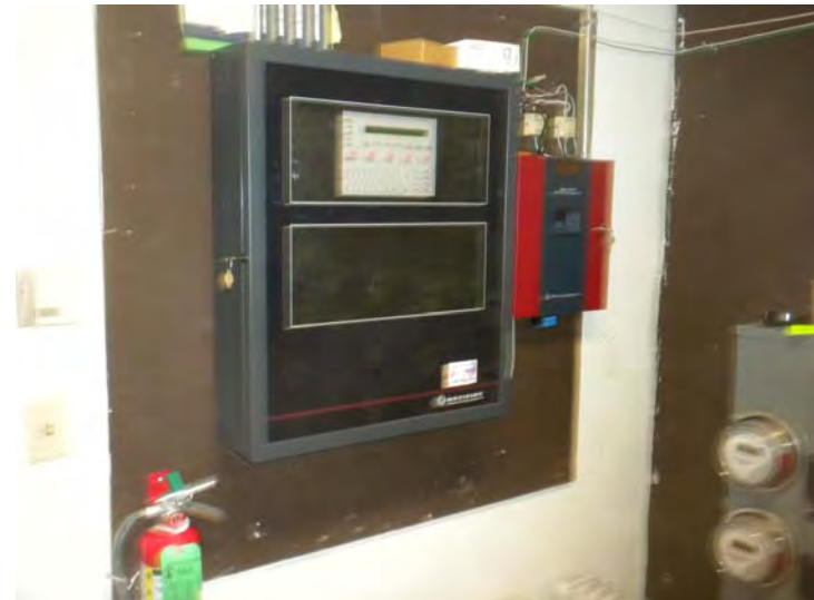
View of the fire alarm control panel
