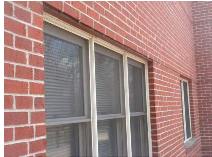
View of a rusted window lintel
